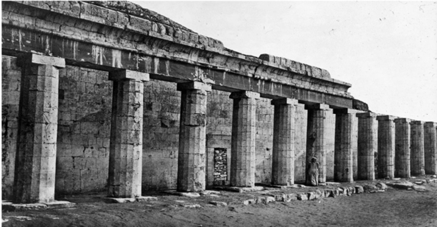
Figure 14. Is showing a group of free standing columns supporting the retaining Wall of the mountain at Deir el-Bahari."Reference: [19].
