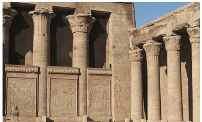
Figure 3. Is showing several Egyptian columns with different architectural crown styles all Assembled in one façade. Image Is that of the Temple of Horus "in Edfu," Egypt. Reference: [7]. 2
