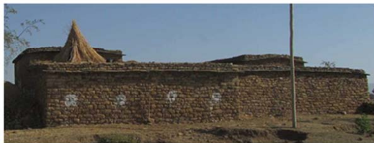
Figure 3. Typical hidmo house.
