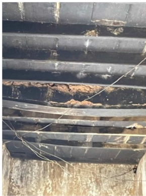
Figure 20. Showing failing first floor support in need of restorative intervention.
