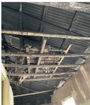
Figure 8. Showing extent of dilapidation in the Ka Esin (Courtyard to stable for horses).
