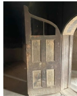
Figure 10. Showing wall thickness, wooden lintel support.
